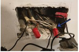
After turning off your breaker, pull out the switches (**WARNING:** there may be multiple circuits in one gang-box -- please ensure all circuits are turned off). Check the back of your gang-box for a bundle of white wires. These are typically neutrals.
